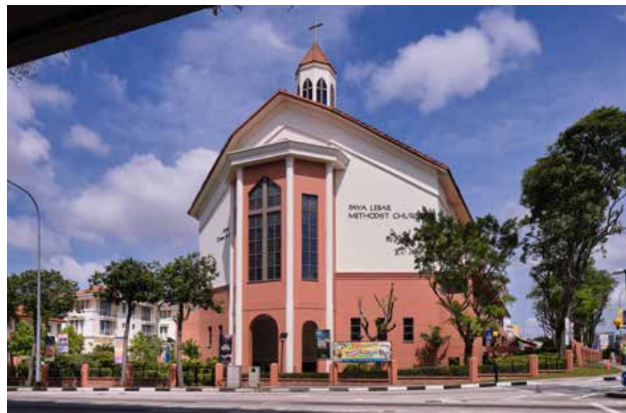
The Paya Lebar Methodist Church, 2020 Courtesy of National Heritage Board
