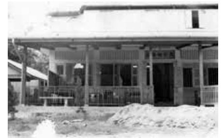
The temple building before it was rebuilt in 1982 Courtesy of Tian Kong & Kancanarama Buddhist Temple
