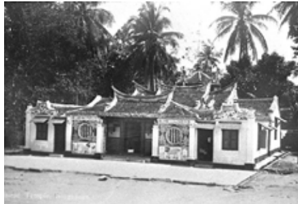
Prior to renovations, the temple's roof ridges were distinctively Hokkien in their pronounced curvatures, c. early 1900s. Courtesy of National Archives of Singapore
