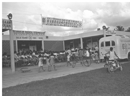
Nee Soon Community Centre and mobile library service, 1965
