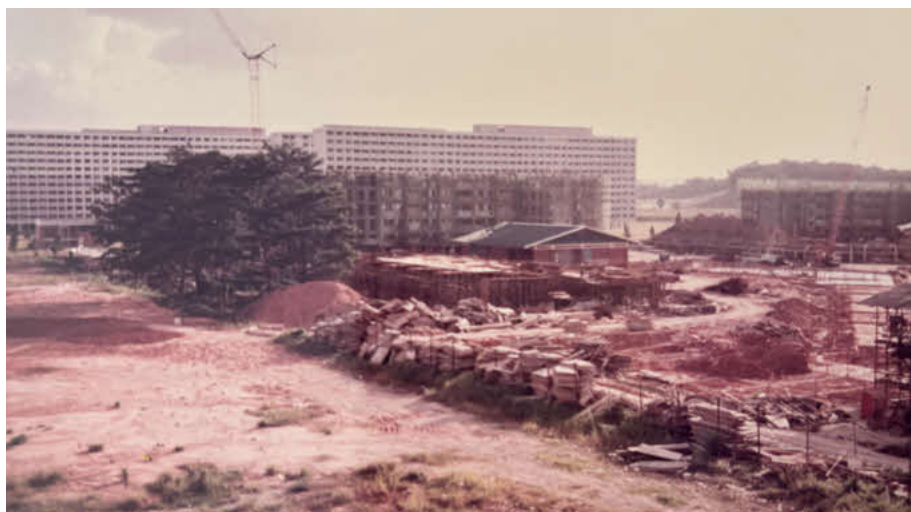
Flats under construction at Yishun, late 1980s Courtesy of Sofea Abdul Rahman
