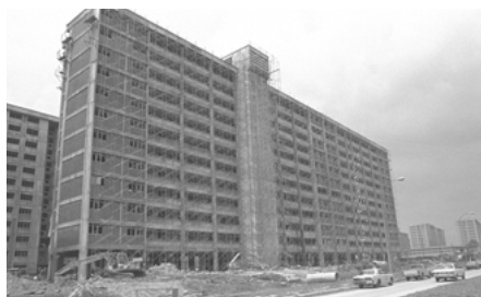
Construction of Yishun HDB flats, 1983
