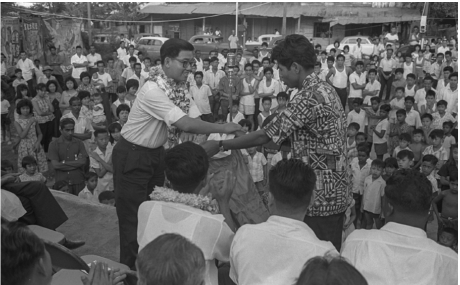
Sembawang Legislative Assembly member Teong Eng Siong officiating at a street lamp opening ceremony at 12 1/2 milestone, Sembawang Road (junction with Chye Kay Road), 1965
