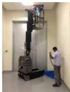
Fig. 2. Cabling installation using existing trunking to avoid intrusive renovation works.
