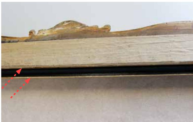
*Fig. 17. Close up image of the polyethylene foam tape and mat board strip on the frame rabbet and lip respectively.*
