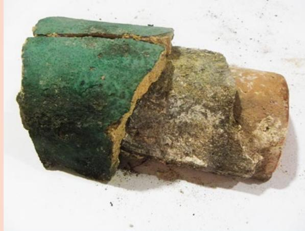
A cross-section of a roof tile of the former Keng Teck Whay Building, showing the original terracotta tile (reddish-brown material). During restoration works in 2012, it was discovered that the tiles were in fact terracotta and not plaster as previously assumed.
