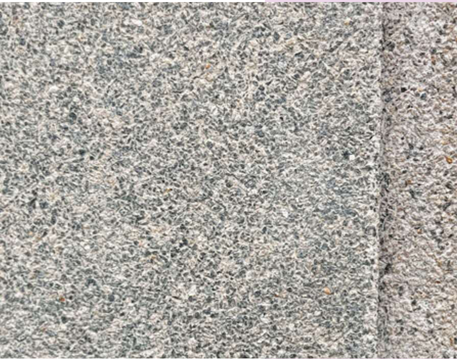
↓ A close-up of Shanghai plaster, which typically employs an aggregate–cement ratio of 2:1. Commonly used aggregates are granite gravel and fine sands. After cladding a building’s facade, water is used to wash the cement binder in order to expose the aggregates.
