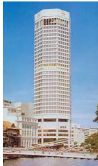
The United Overseas Bank (UOB) Building, 1970s-80s
