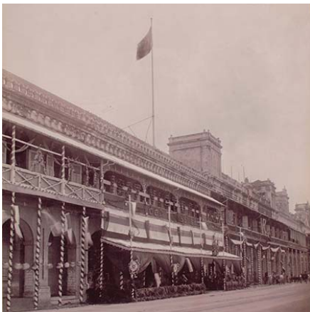
The Guthrie and Co. offices at Collyer Quay, established by Alexander Guthrie to deal with import of British manufactures and Straits produce, as well as insurance, 1897
