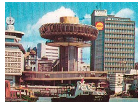
Change Alley Aerial Plaza along the Collyer Quay waterfront, c. 1974
