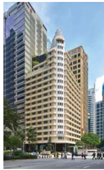
Former Asia Insurance building (now Ascott Raffles Place), 2016
