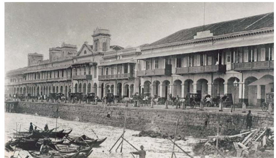
Office buildings and godowns along Collyer Quay, c. 1880s
