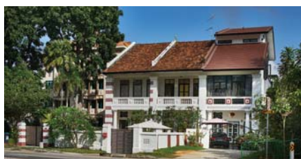
A row of Neo-Georgian style shophouses along Upper East Coast Road, 2016
