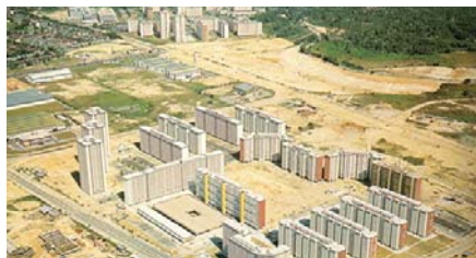
An aerial view showing Bedok New Town, Neighbourhood 1 with 4,000 housing units, and Chai Chee Estate in the background, 1974
