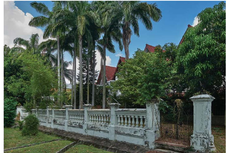
A now-landlocked seawall near Marine Parade Road, 2016
