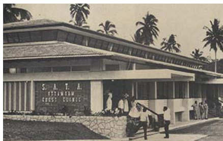
The Uttamram Chest Clinic on the year of its opening (now SATA CommHealth Uttamram, Bedok), 1962
