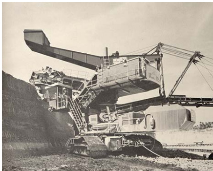
A bucket wheel excavator cutting earth for land reclamation at Bedok, 1966
