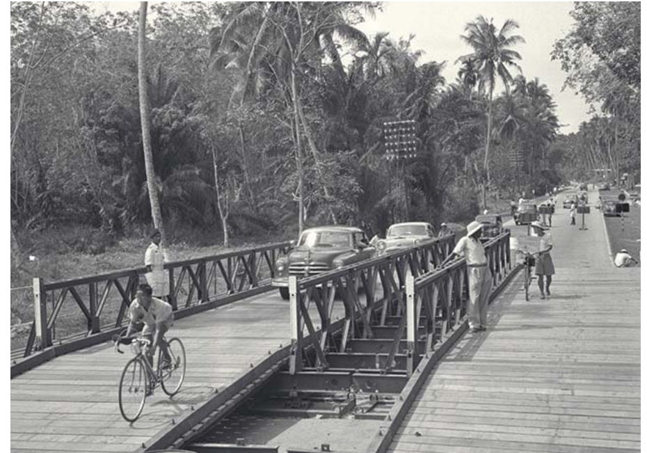
The Bailey bridge at Bedok settlement, 1955
